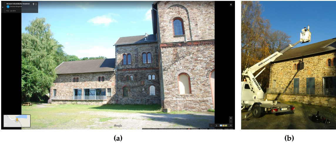
Figure 5.44: Photograph of the Haseschacht headframe building (a) and of scan acquisition (b). Photograph (a) taken by Christian Bergstedt and published on https://www.google.de/maps , use in accordance to Google’s permission guidelines and “Fair Use” policy.
