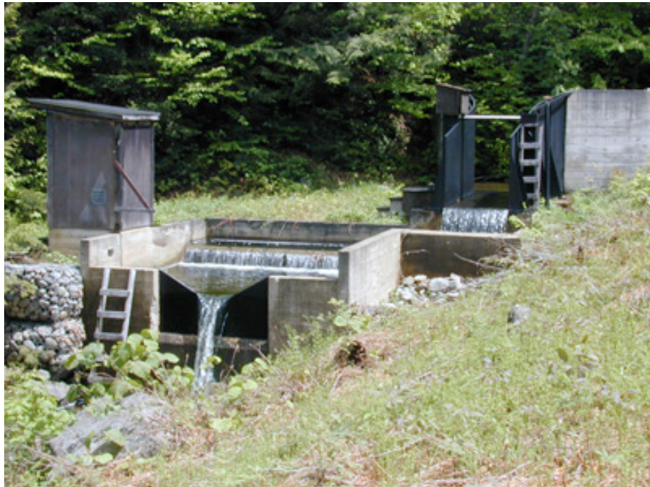
Figure 6. Triangular weir.
