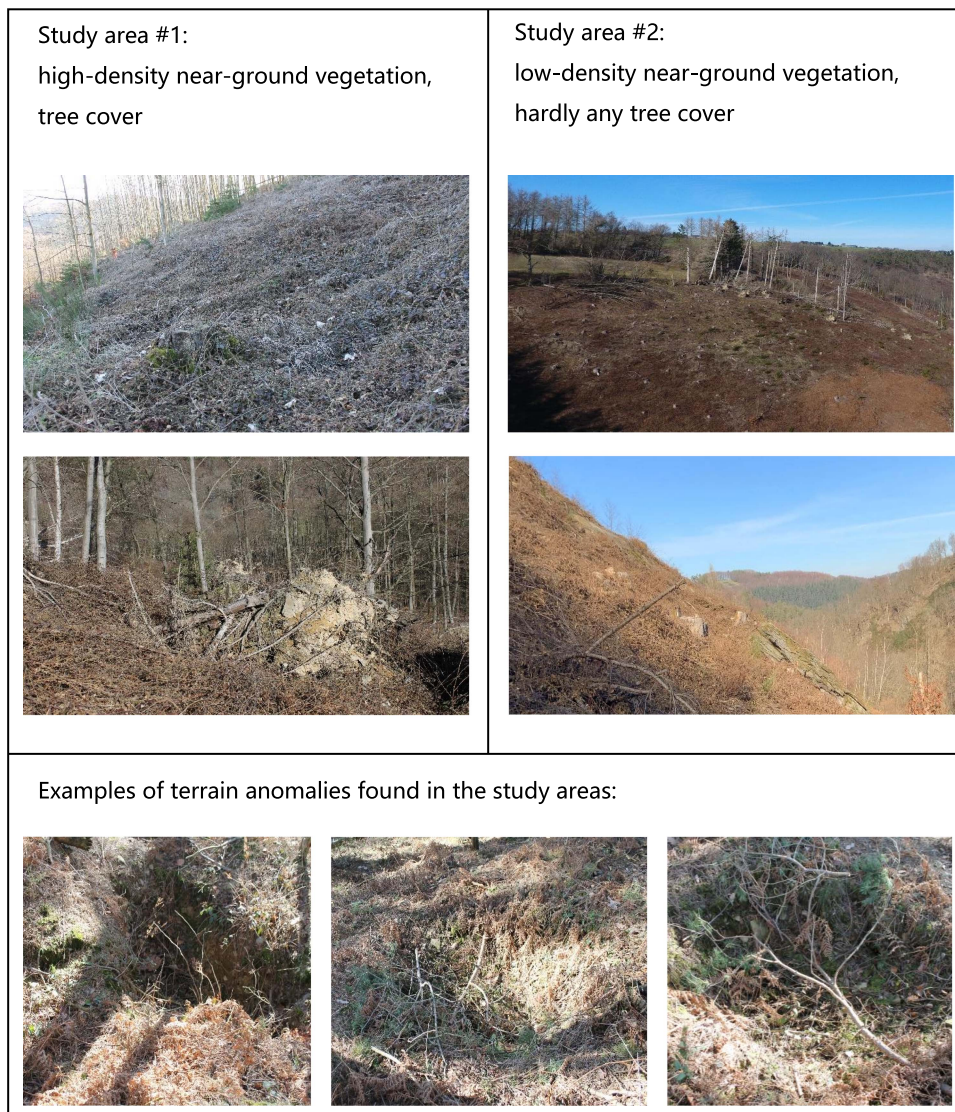
Fig. 2. Photos of the research area (photos taken on March 6, 2021 by M. Adam, M. Storch).
